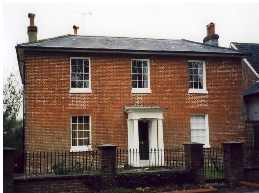
Bourne House from the Georgian era
